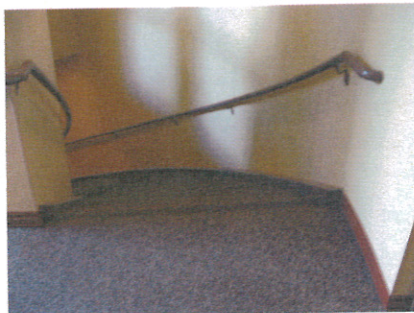
Inside of Interior Stairwell
