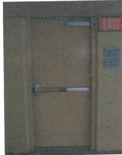
Exit Door to North Side Exterior Stairwell
