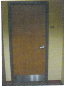
Entrance to Stairwell
